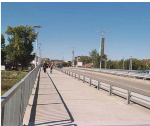
Pedestrians and drivers in the northwestern Bulgarian city of Montana now enjoy an improved and better-lit road connecting the city to the main highway.
