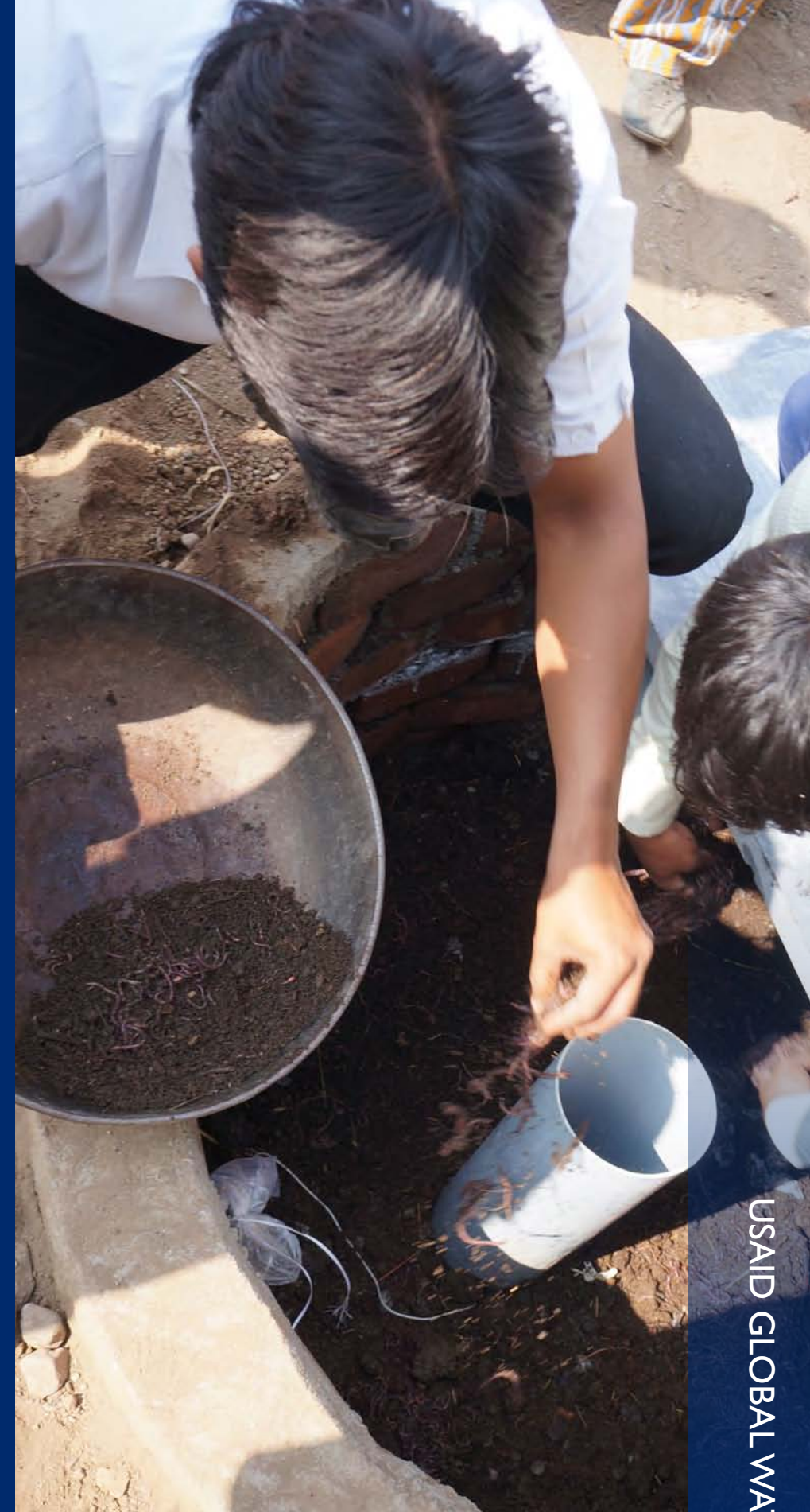
SUSTAINABLE SANITATION: The Tiger Toilets are new latrines which contain worms that eat excrement, reducing the system's waste by more than 80 percent.
