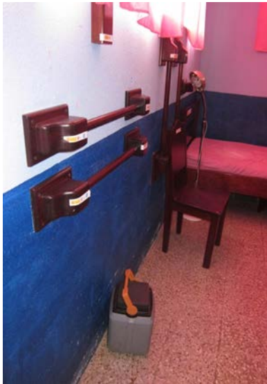
FIGURE 5.9. HANDRAILS IN INTERCULTURAL VERTICAL BIRTHING ROOM
