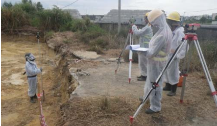
Verifying excavation depths (Photo: CDM Smith)
