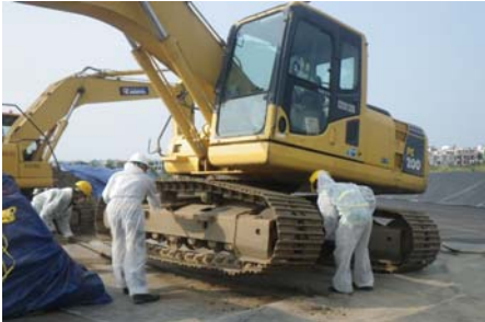
Equipment decontamination (Photo: CDM Smith)
