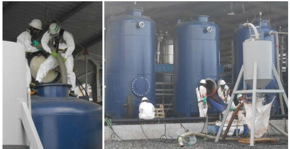
Changing out carbon media in the liquid treatment vessels
