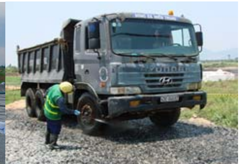
Washing truck tires to prevent contamination from leaving the project site (Photo: TetraTech)
