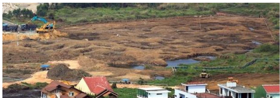
Excavation in the wetland area
