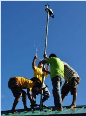
Automated Early Warning Systems were installed along with Automated Weather Stations (AWS). The AWS monitor a range of meteorological data, such as barometric pressure, rain fall, rain rate, temperature and humidity. (Photo: WFP Philippines)
