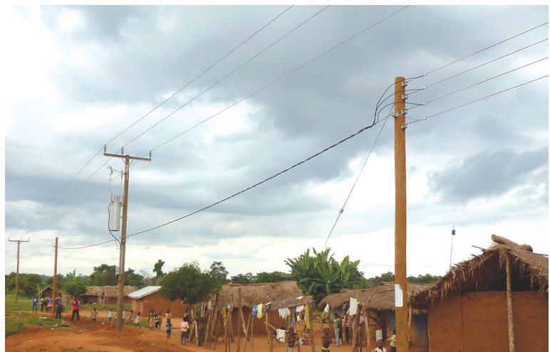
Distribution lines running to a village in the Brong Ahafo region of Ghana. Photo: Weldy Lamont Associates, Inc.
